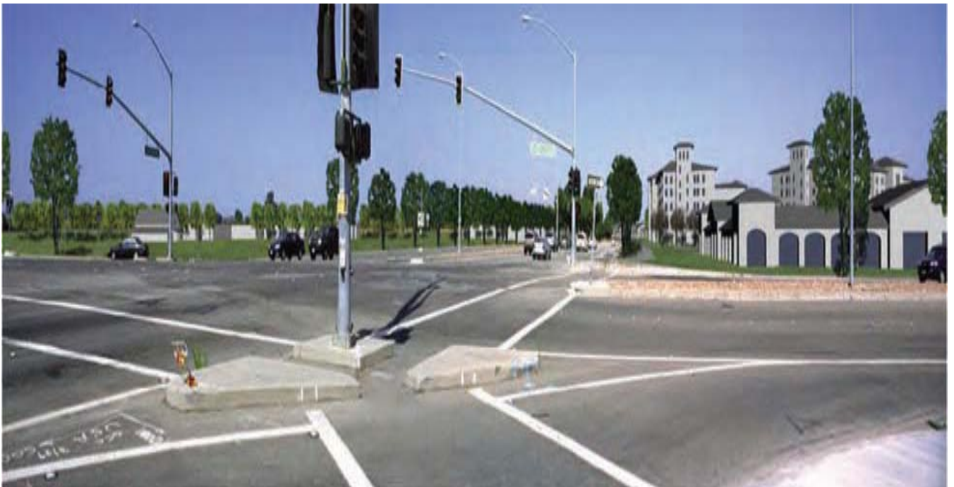
Paseo Padre Parkway and Ardenwood Blvd: 5-story buildings and strip mall, blocking view Coyote Hills. Housing units and retail space built on soils at high risk of liquefaction in an earthquake. Convenience store open 24/7 would bring traffic, crimes, noise, and alcohol to neighborhoods and Coyote Hills park.
