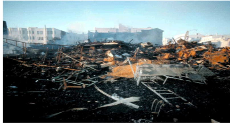
SF Marina district, Loma Prieta earthquake: Homes built on liquefied soil
